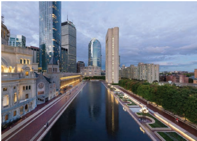
The First Church of Christ, Scientist, Boston - MA, renovation of plaza (built in 1970)
