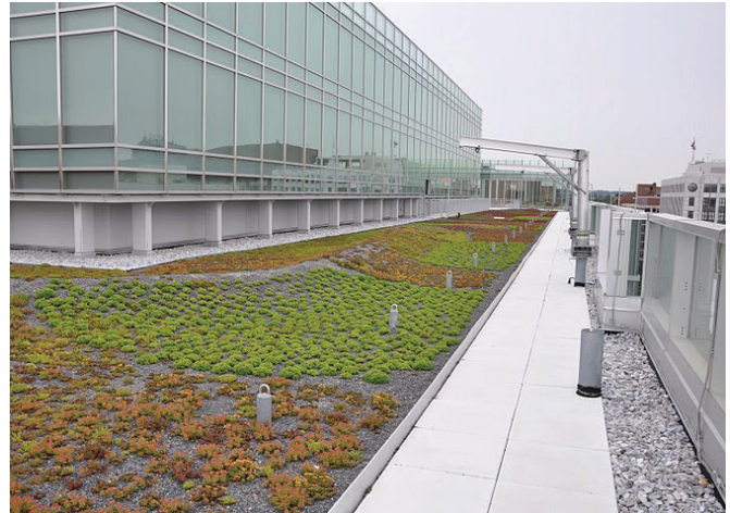
1225 Connecticut Ave - Washington, DC - renovation of roof deck, (built in 1960, renovated 2008)
